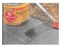
Step 2- Apply the QuickPrime™ Plus Primer several inches (approximately 7.62 cm) down into the anchor trench.
